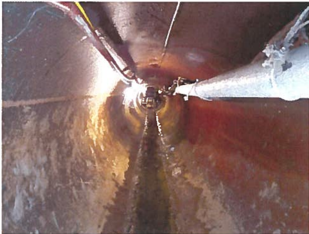
Looking upstream at rear of Tunnel Boring Machine
