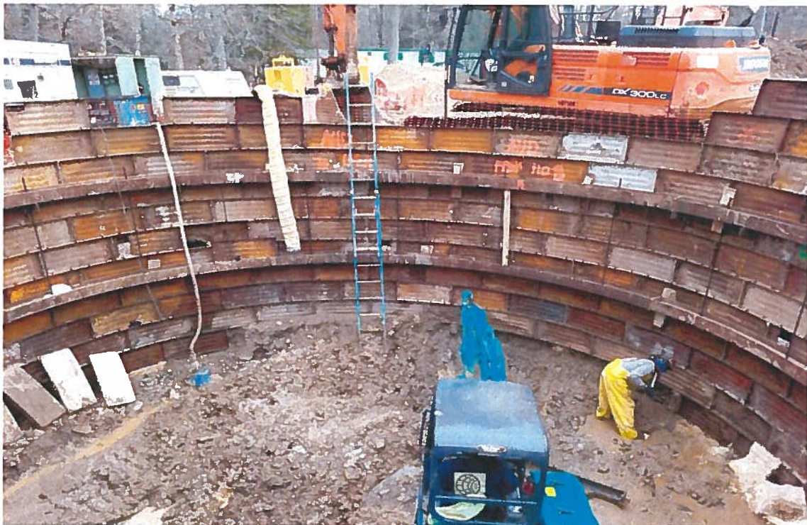
Microtunnelling/Boring Shaft Construction
